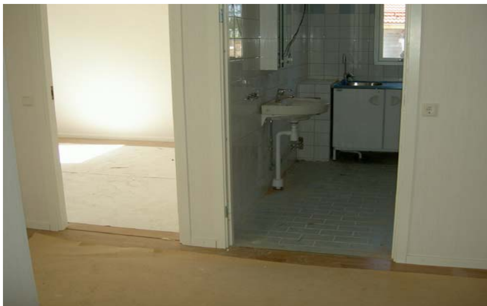
figur 51. Extra bred badrumsdörr (1 meter)
